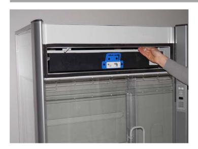
Using the handle on the front of the filter casing, pull the filter outwards away from its housing. Important – the filter is heavy and two people will be needed to take the weight and lower the filter.
